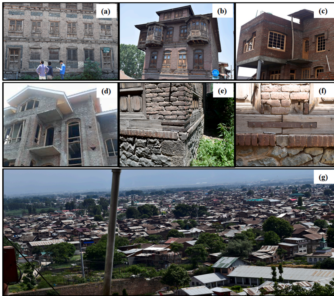
Fig. 14. Building practices performed in the Kashmir valley. The traditional construction include (a) Dajji Dewar (b) Taq system, the present unsafe structures are depicted by (c) and (d), (e) and (f) shows the wood runners at floor level and connection of bracers, (g) represent the density of settlement at Srinagar city.
